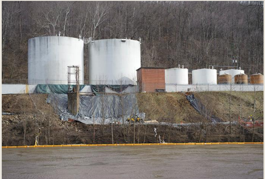
Leaking Tanks from Elk River Spill
