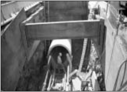
A new line is installed as part of a sewer system separation project in New Brunswick, New Jersey.
