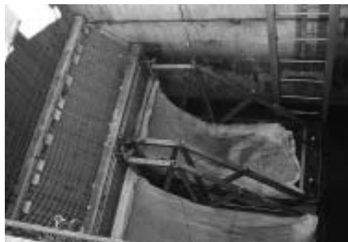
Photo: Solids and floatables controls, such as the nets pictured here, are installed at all North Bergen CSOs.
