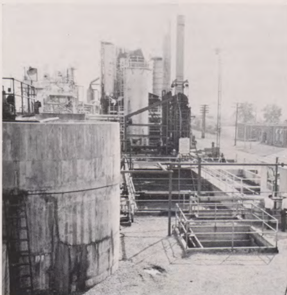
Oil-waste treatment plant built by the Rock Island Refinery Corporation at New Augusta, Indiana. At left is a flocculation tank; oil separator tanks are shown in center, and chemical treatment house at right.
