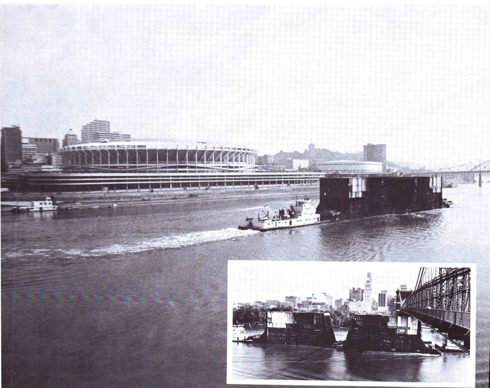
A tow guides a power plant up the river toward the new hydroelectric facility at Greenup Dam
