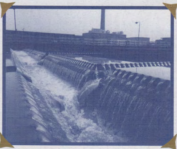
Waste water treatment facility located along the Ohio River
