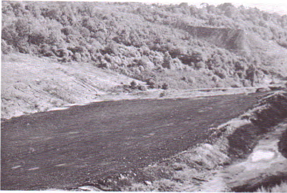
Coal refuse disposal showing drainway to carry surface water around refuse pile.
