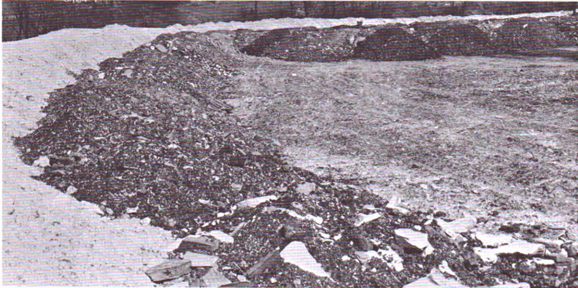
Coal refuse disposal showing coal refuse deposited behind a clay face wall and on top of a previously deposited layer of coal refuse which has been leveled and thoroughly compacted by the directed travel of refuse trucks.
