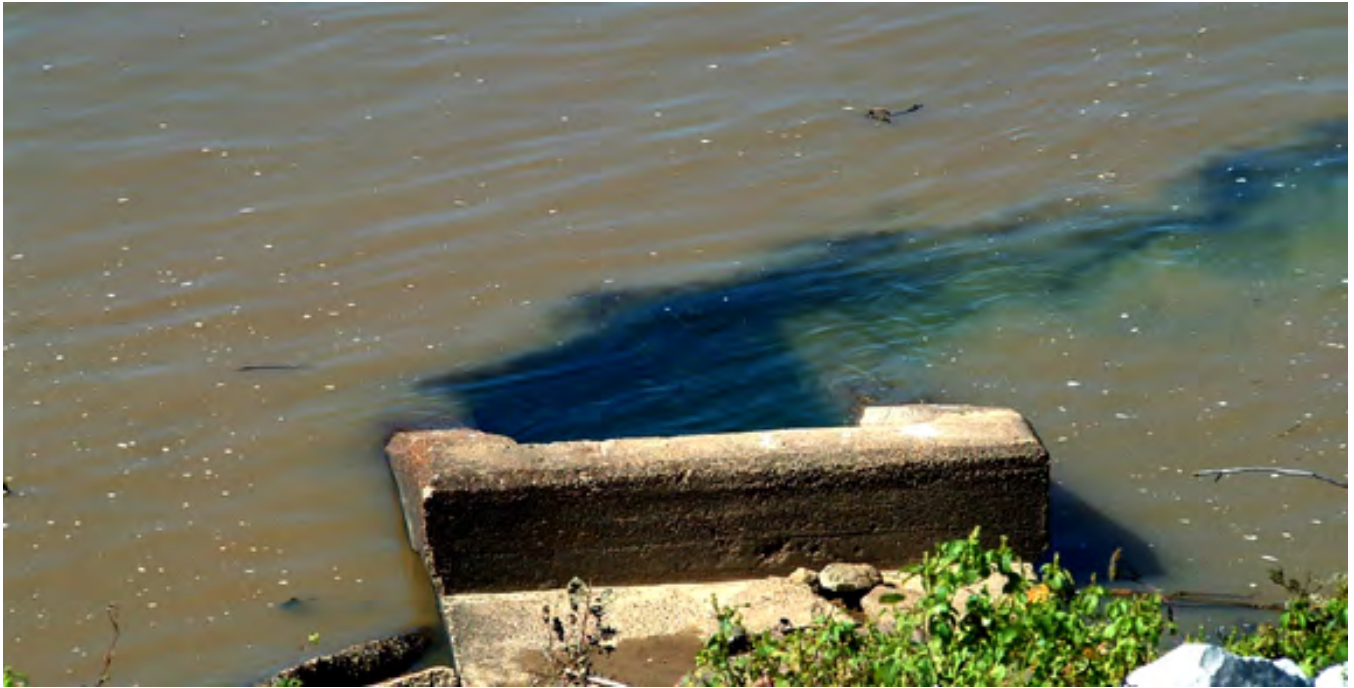
Some municipal sewage at Evansville
